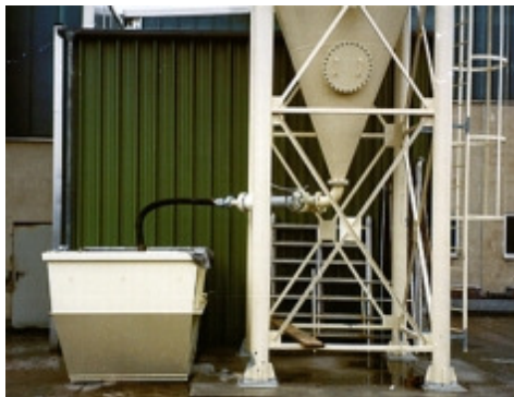
ECON container to drain sludge; capacity: 1,5 - 9 m 3 .
